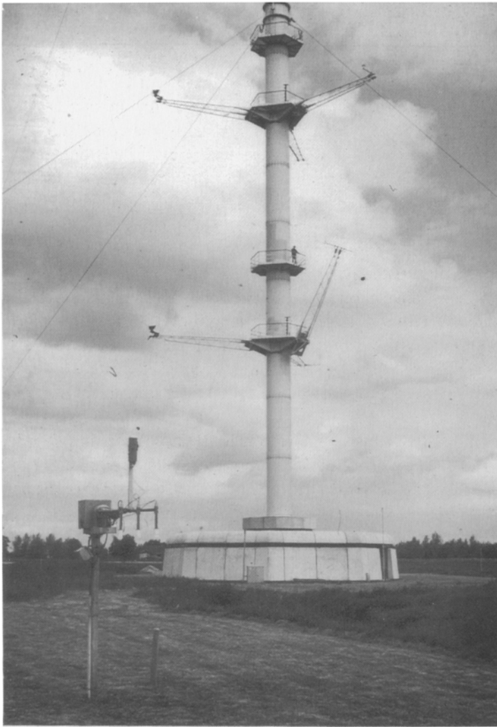
Figure 2. Raising a boom on the Cabauw mast.
