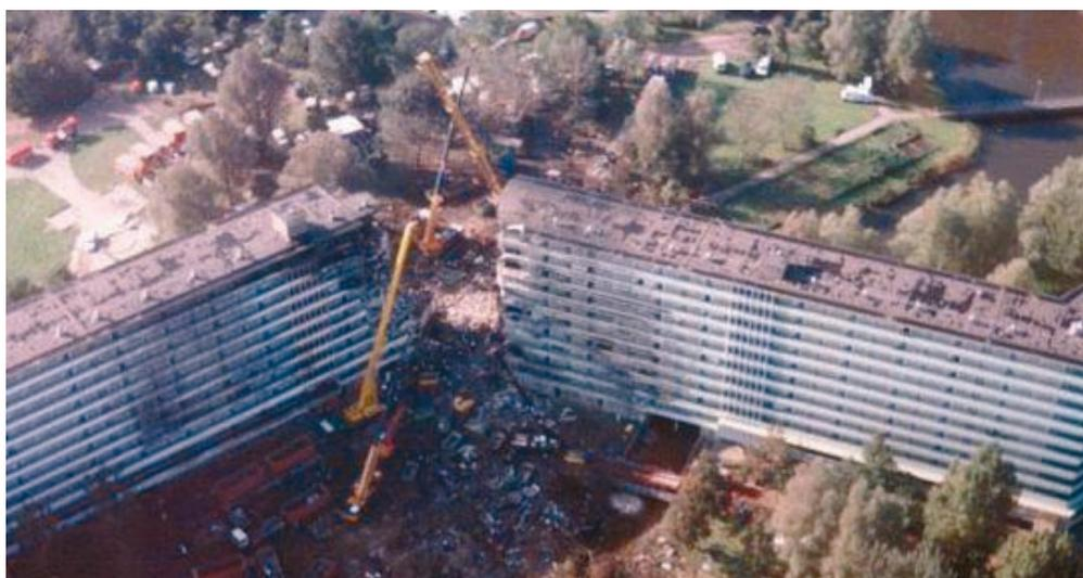
Figure 23: Apartment building after being hit by a Boeing 747 Amsterdam "Bijlmer", October 4th, 1992.
