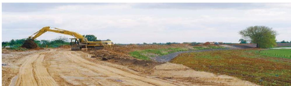
Figure 43 Widening and heightening of a dike
