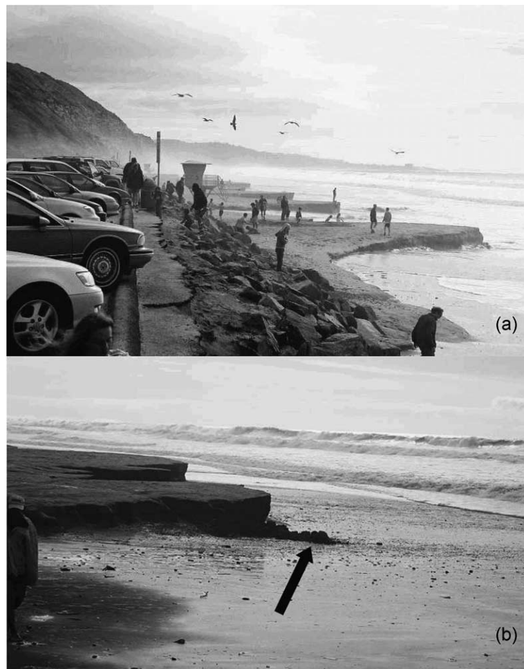
Fig. 8. Photographs (looking south) at the storm peak (1300 PST, 22 November 2001) showing (a) erosion occurred as a series of embayments and (b) steep-faced scarps eroded by slumping (indicated with an arrow) that was visible during wave downwash.
