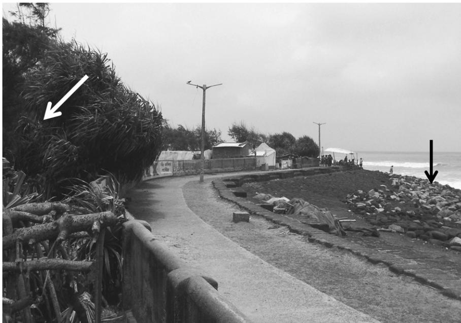
Fig. 5. Seawall within LC3 with artificial mangrove plantation (white arrow) and boulders along beach (black arrow), as efficient barrier against coastal flooding and beach erosion.
