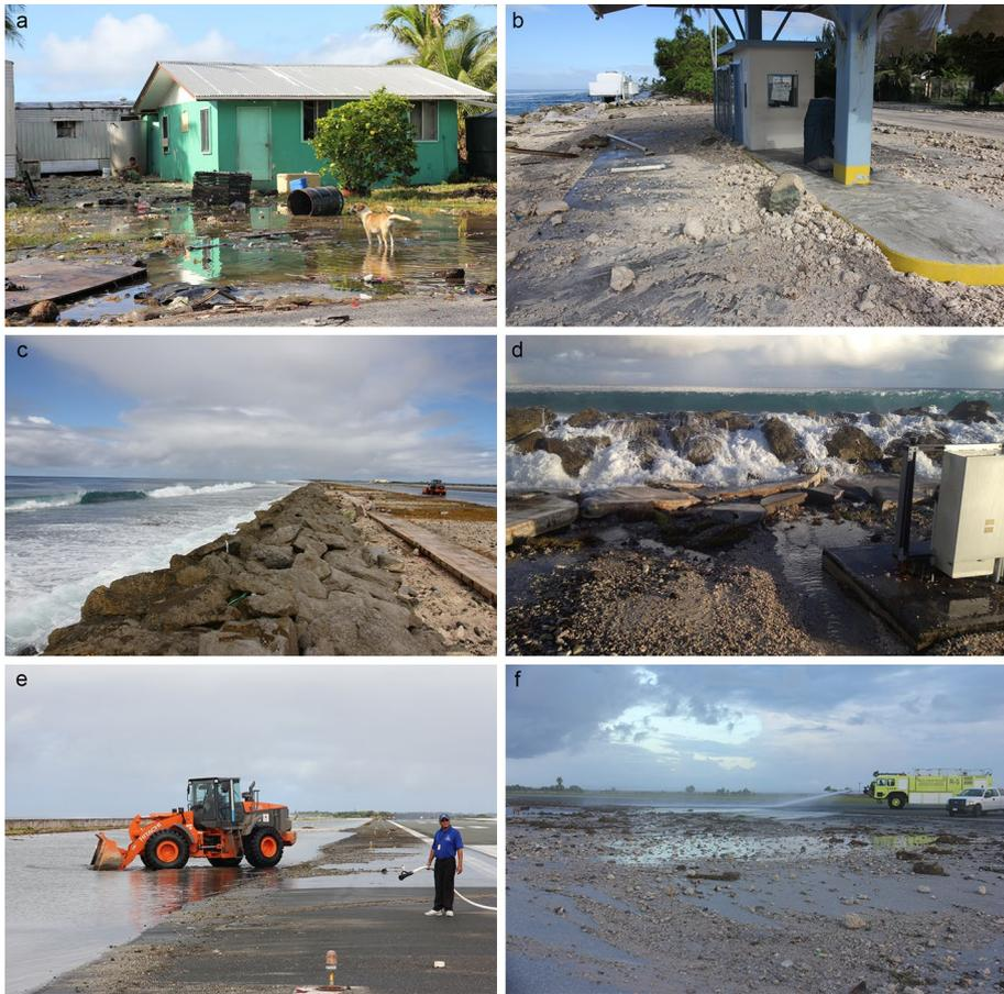
**Fig. 9** Impacts of the 25 June 2013 wave-driven inundation event: **a** ponded water and mix of organic and inorganic debris deposits on southern Majuro, **b** sand, gravel and coral boulders deposited on sections of southern Majuro, **c–f** damages to coastal protections and subsequent inundation and debris deposition at Majuro International Airport
