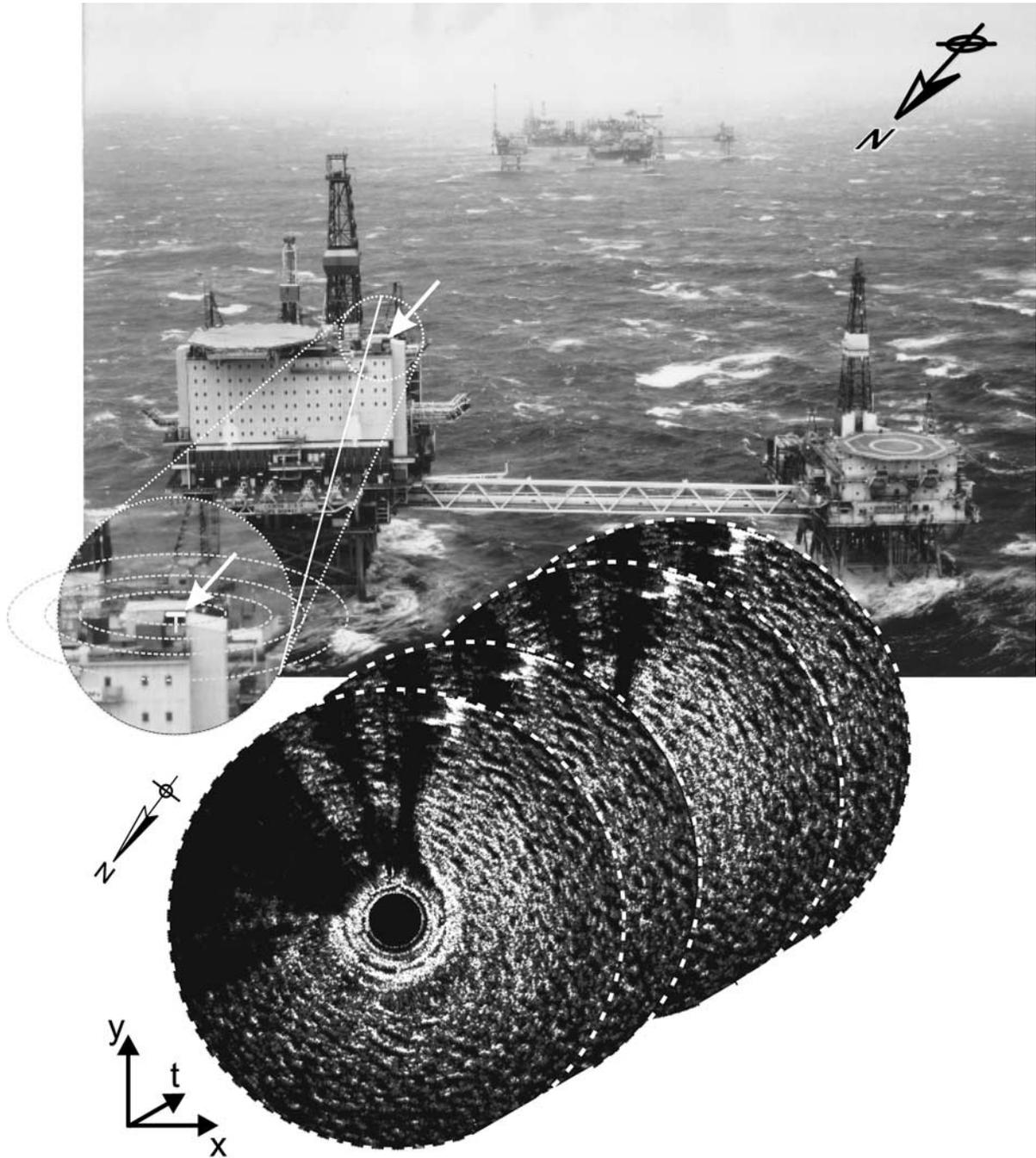
**Figure 1.** Ekofisk 2/4 k platform of the Ekofisk oil field in the North Sea. The WaMoS system is installed at the northwest corner of the platform. In the radar images, several shadows are visible, which are due to the equipment of the platform. The large backscatter in the south originates from the oil field visible in the background of the photo.
