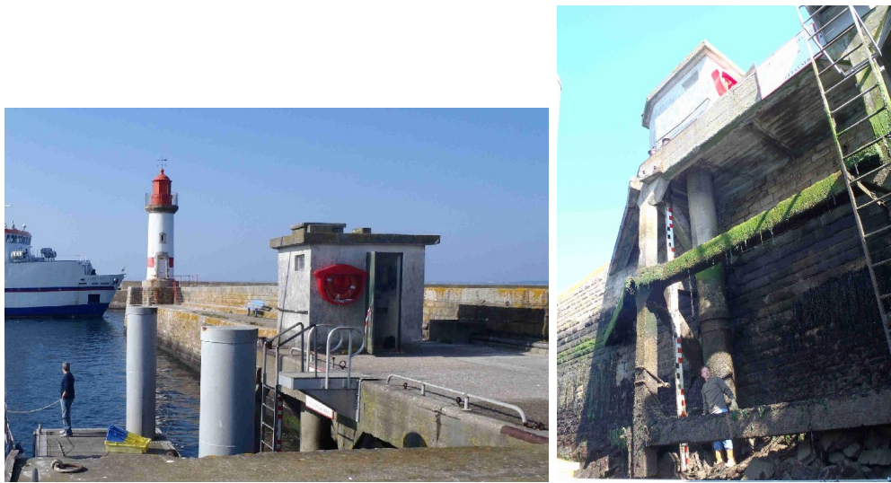
Figure 4.3: Tide gauge installation in Groix harbor. Tide gauge hut (on the left photo) and well stilling (on the right photo).
