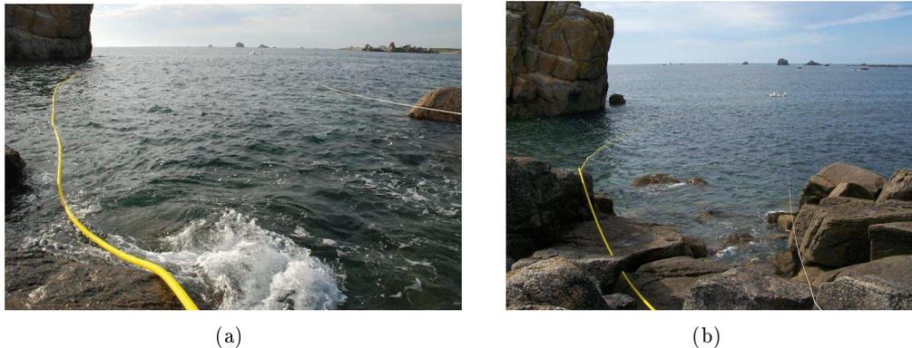
Figure 1.11: The cable with its yellow sheath (a) when the sea is high (b) when the sea is low with a lot of rocks
